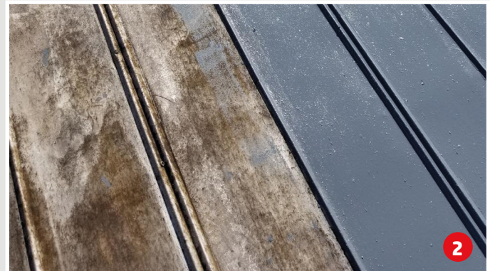
Left side: after applying the FRC, right side after applying FEP over FRC
